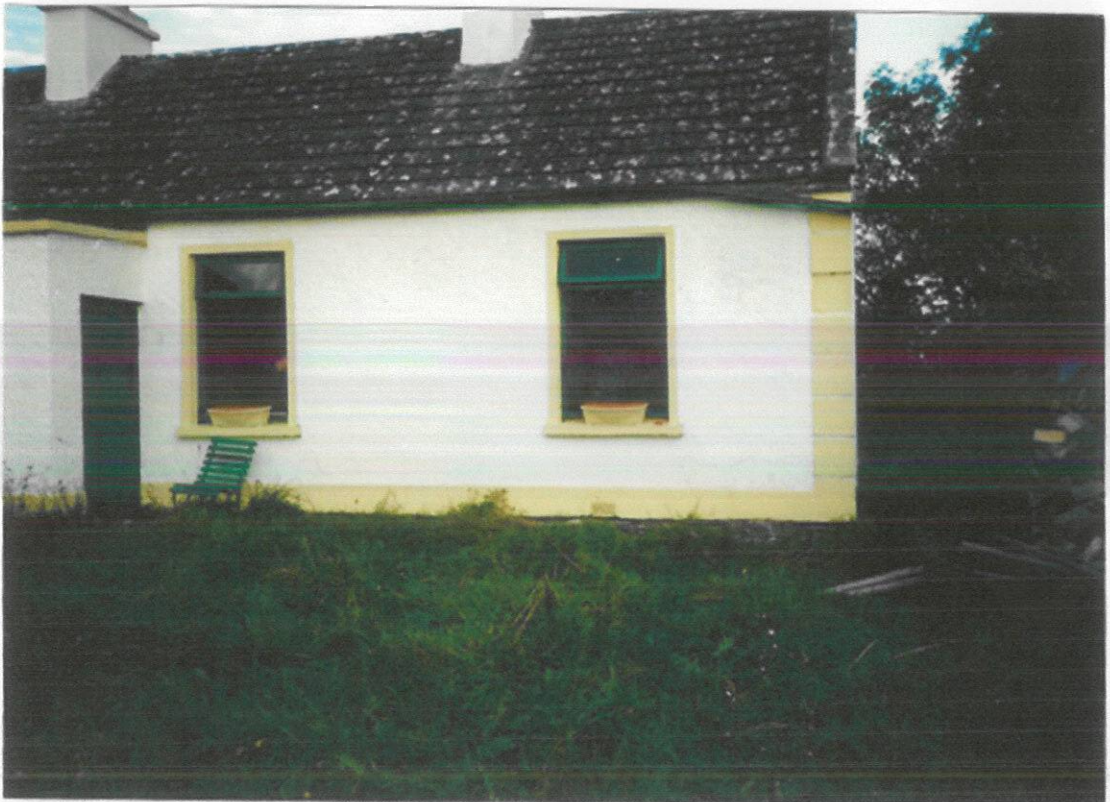
Image of existing dwelling entrance and window detail- approx date photo was taken 1996
