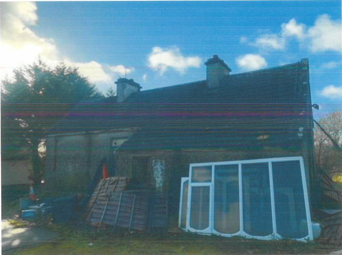
Recent condition image (2021) of rear elevation.
