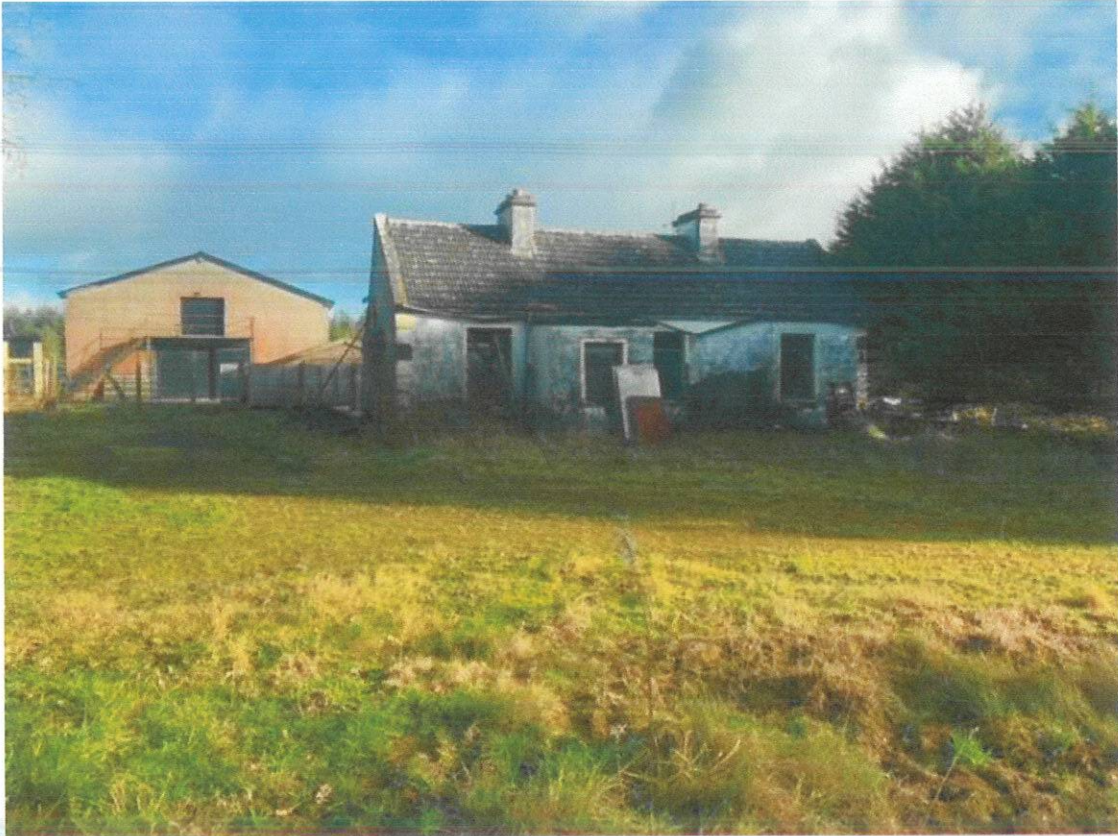
Recent condition image (2021) of front elevation from existing entrance.
